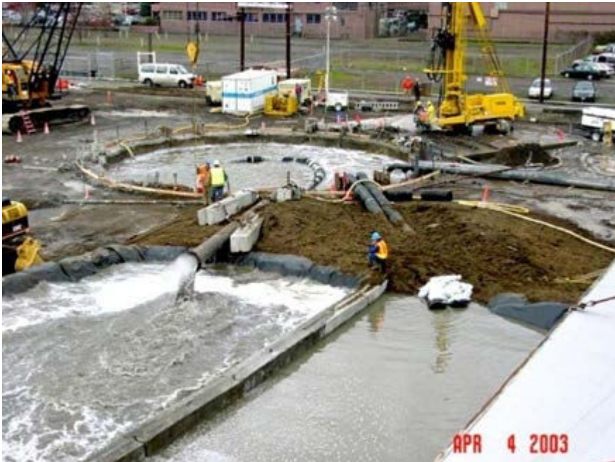
14 #R-88 Couplings for Coarse (abrasive) Slurry outflow
