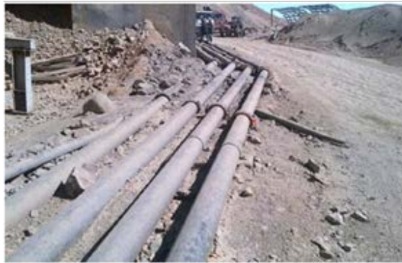
Shurjoint #RX-3000 8" Ring Joint Coupling
