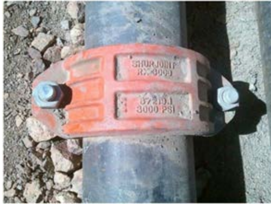
Shurjoint #RX-3000 8" Ring Joint Coupling
