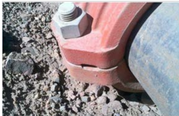
Tighten bolts and nuts until bolt pads make metal to metal contact. No torque wrench is required.
