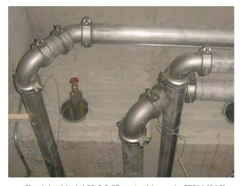
Shurjoint Model SS-8 2.5" austenitic grade CF8M (316) stainless steel couplings were selected and specified in the glycol pipeline because of their cost, quality, durability and ease of maintenance. In addition, Shurjoint #SS-8 Couplings are UL listed and FM approved.
