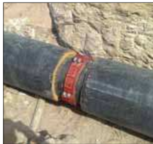
A 28" R-88 coupling installed in a chilled water system.
