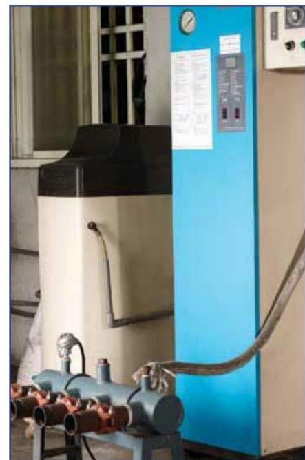
Laboratory hot water testing
